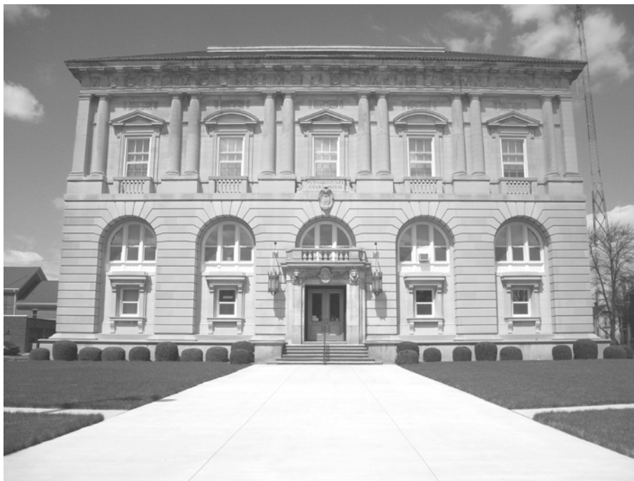
Putnam County Courthouse - Ottawa, Ohio
