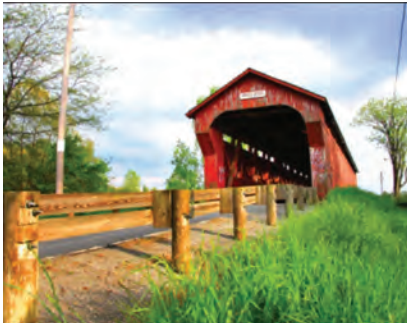
Swartz Bridge, Wyandot County, Ohio
